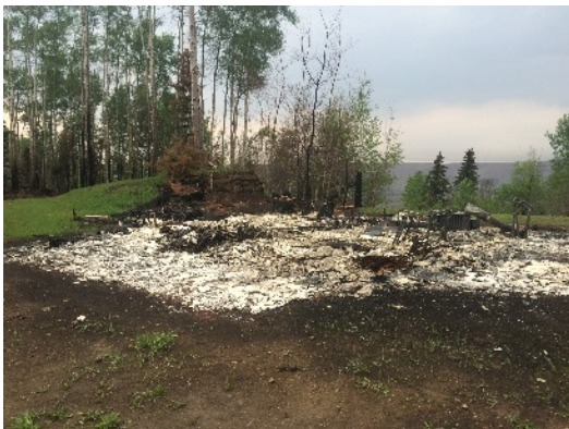
Building destroyed by fire
