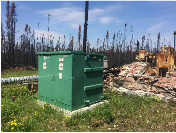
Pumphouse transformer not touched
