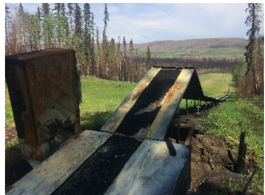
Tube Park lift 600 foot conveyor
