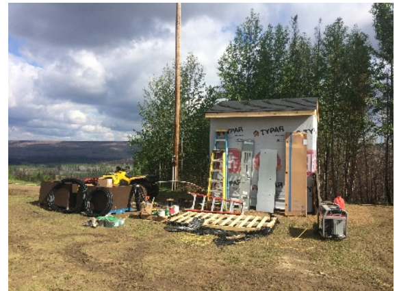
Erecting new hut
